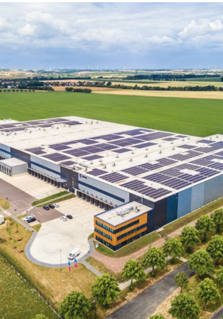
Sustainability: With the construction of its new logistics centres, FIEGE aims to meet the highest standards of the German Sustainable Building Council (DGNB) – as was also the case in Barleben, which is one of the most sustainable healthcare logistics centres in all of Germany.
