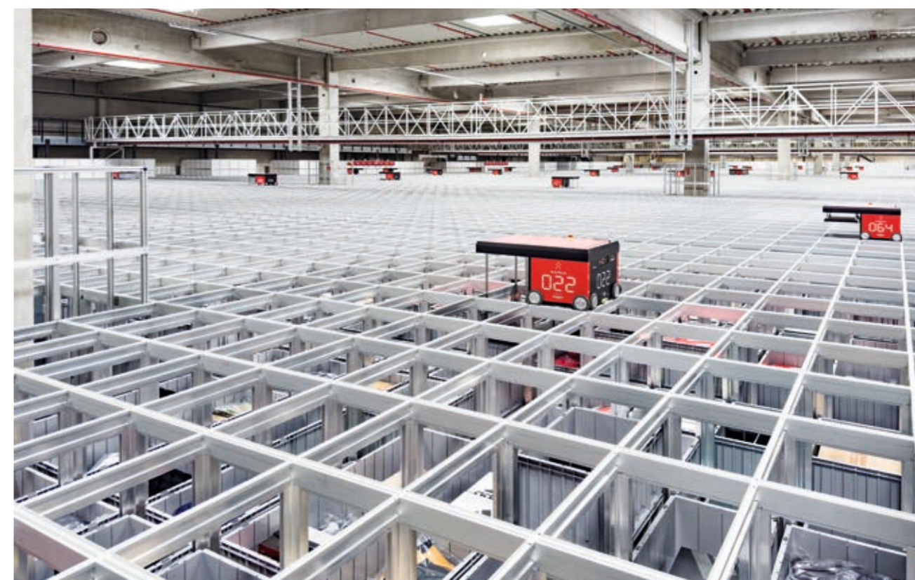
Pioneering: FIEGE built one of Germany's biggest AutoStores for SportScheck at its facility in Apfelstädt near Erfurt.
